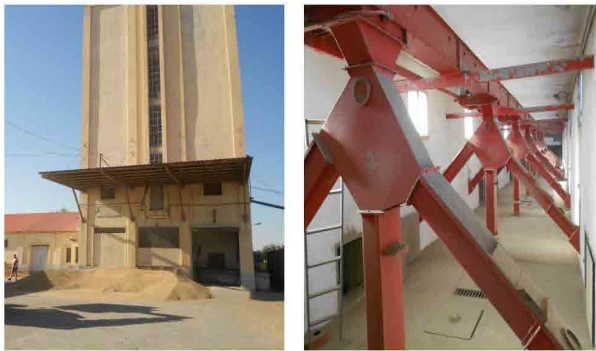
Figure 3: Detail of hopper area and upper horizontal belt conveyor and distribution tubes in D5 silo at Manganeses de la Lampreana, Zamora.
