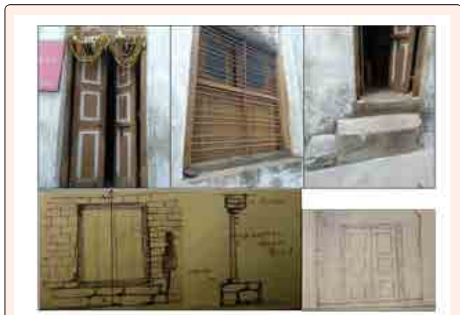
Figure 8: Shows the entry of the residence that is fixed up with teak wood double panelled framed door below brick lintel with low height opening size of 0.90m X 1.80m. The style of doors and windows used were those as used in wadas with raised plinth, brick lintel with very less or no ornamentation.
