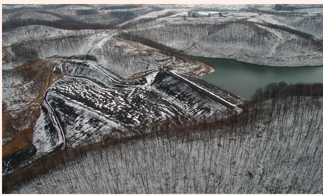
Figure 1: Aerial view of a coal mine waste slurry impoundment. The embankment across the valley is built with coarse coal wastes from mining to create a fine coal waste collection pond. Water from the preparation plant near the coal silos on the hill transporting fine slurry is decanted in the pond below. Adopted from [5].
